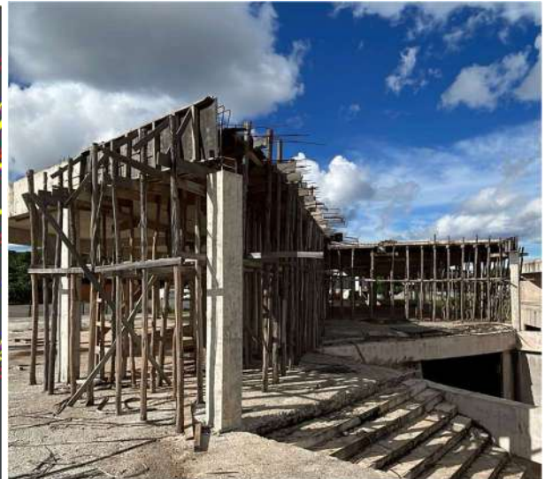
Figura 30: Concreto – Bloco B
